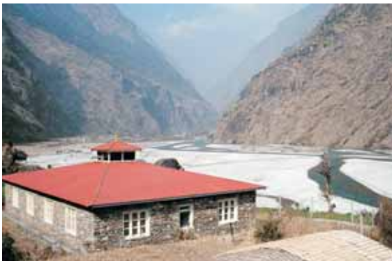
Upper Tamakoshi Project Site
