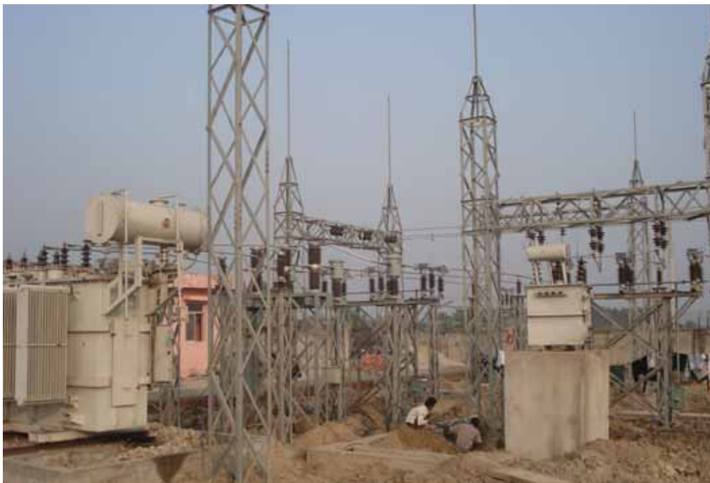
Construction of 33/11 kV Substation at Aurahi
