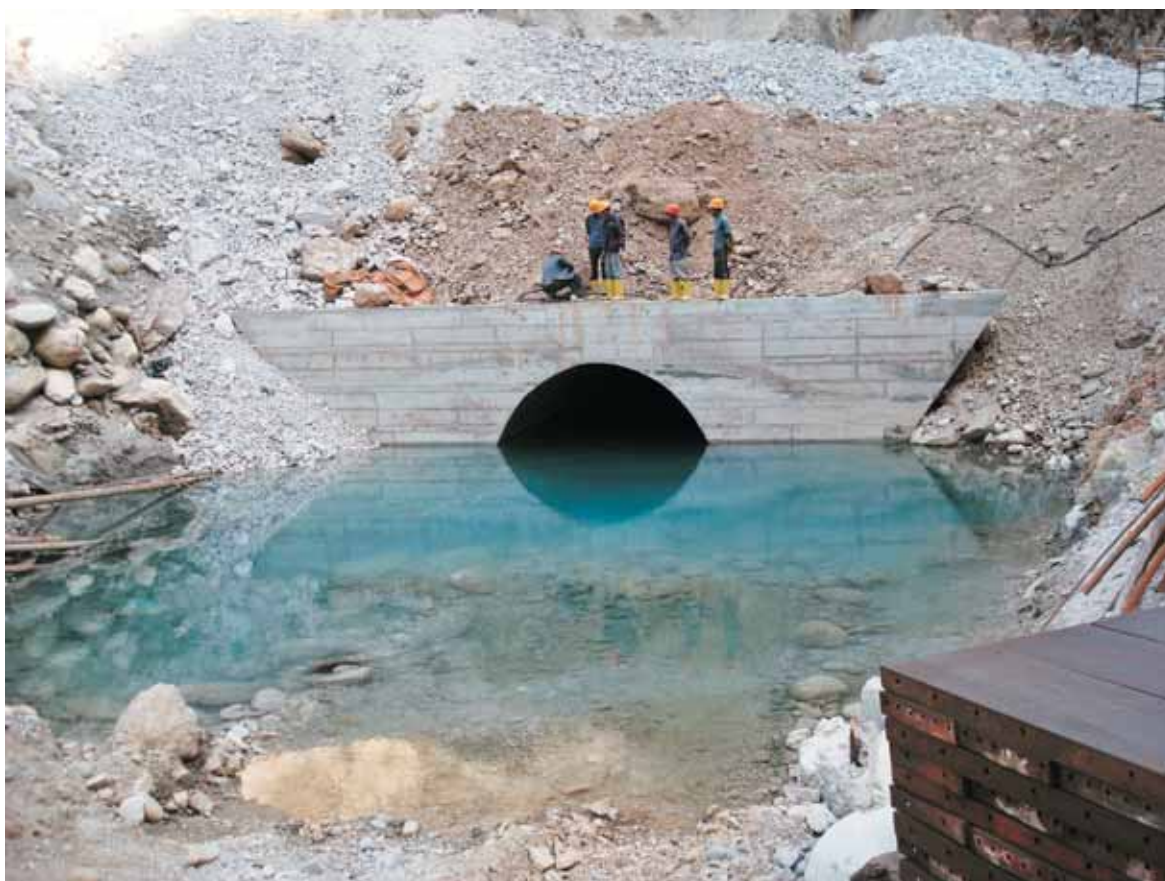
Flushing Tunnel of Chameliya HEP
