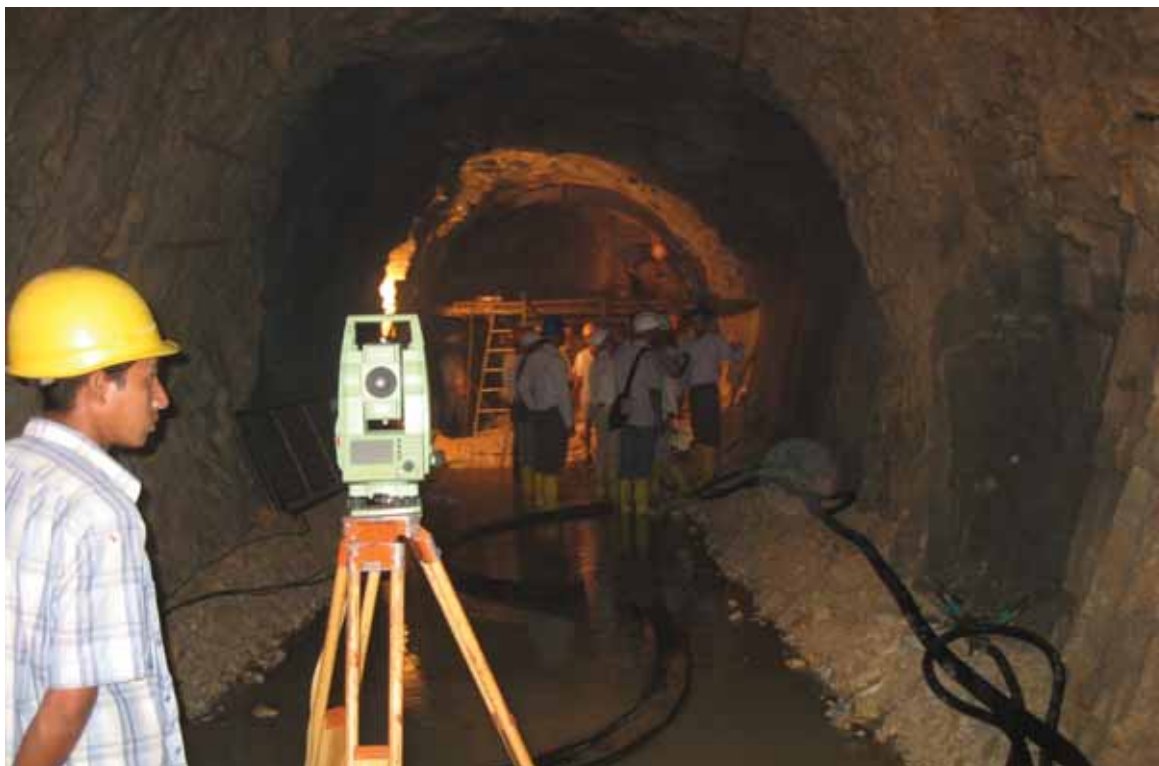
Tunnel Construction of Kulekhani III HEP
