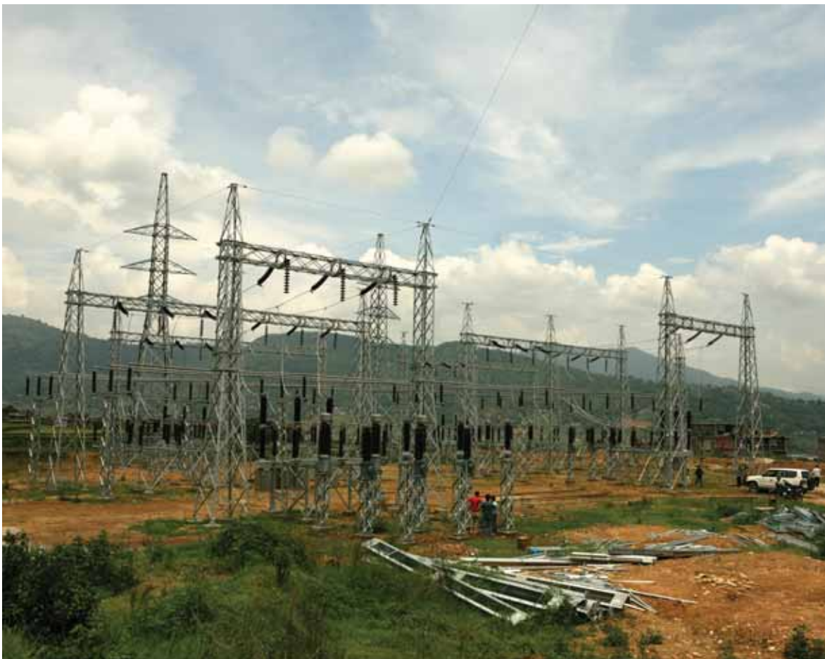
132 kV Matatirtha substation under construction
