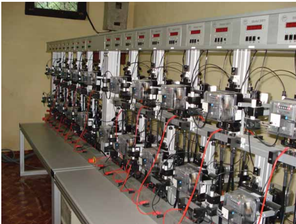
Meter Testing Bench installed by REDSRP at NEA Office, Hetauda
